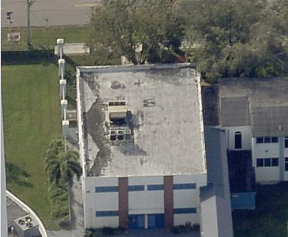
North Side View
