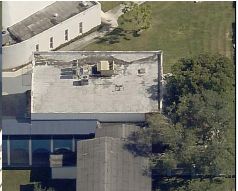
West Side View
